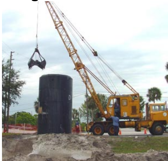
New wet well is trimmed in as part of the project.
