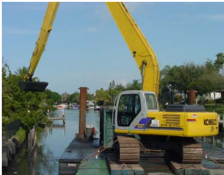
Muck being dredged from the Rio Lindo canal.
