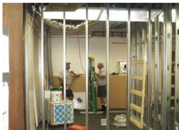
Electricians Greg Valenti (left) and Don DeLoach perform occupant safety evaluations.
