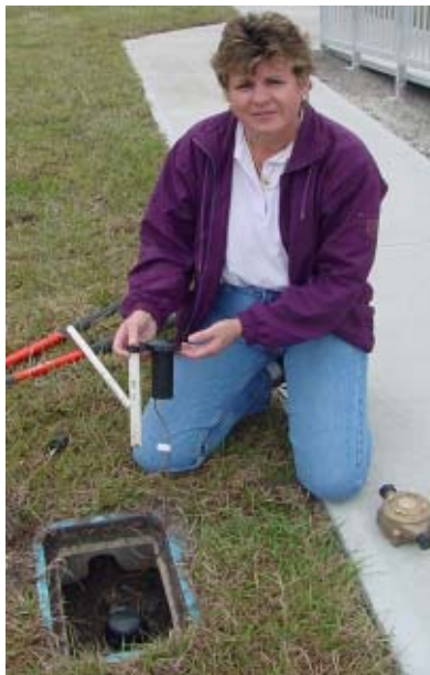
Patti Cheary holds the transmitter unit for one of the new meters.
