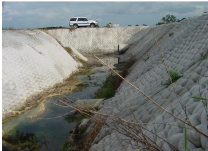
Fabri-Form lines drainage ditch in Eagle Lakes subdivision.
