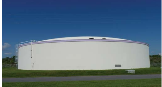
Pictured is the new 2 million gallon storage tank.
