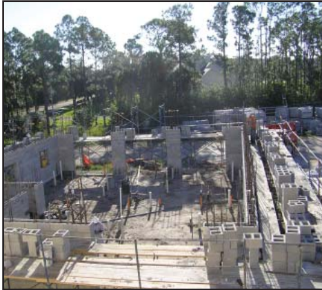
Ozone generator building
