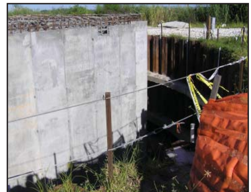
Raw water pump station.
