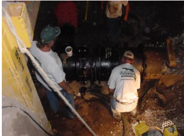
Workers with Florida Design Contractors work on the tie-in.
