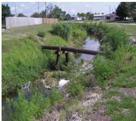
Wastewater pipe over Bell Street ditch.
