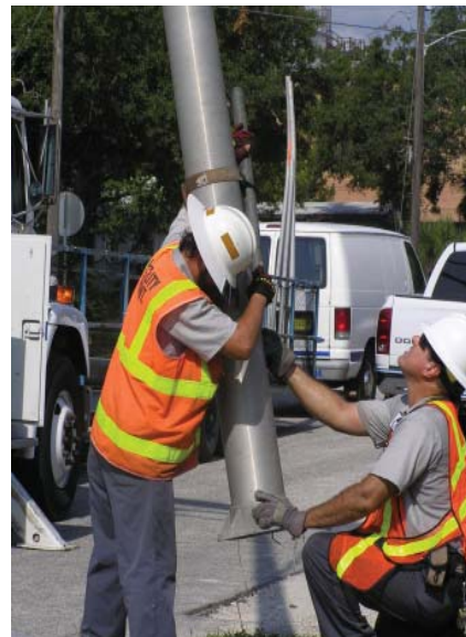
Jim Nickelson and Kurt George guide street light into place.
