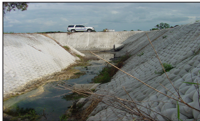
Fabri-form is used to stabilize a City canal.
