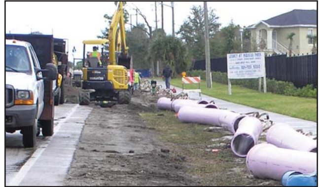
Pipe ready for installation along Airport Boulevard.
