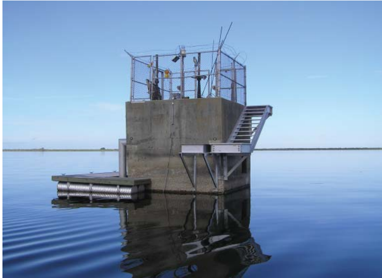
South raw water intake structure on Lake Washington.
