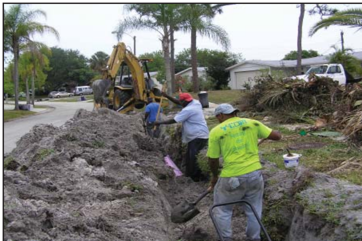
Workers from Y-Com install new reclaimed water lines on Caribbean Drive.
