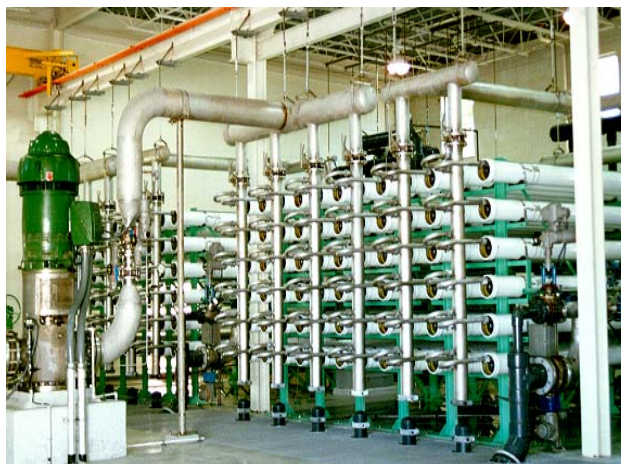
Shown to the left are the membrane trains used to treat water obtained from the Floridan Aquifer wells. The peak capacity of the RO plant is 6.5 MGD. Work is in progress to expand the plant capacity.
