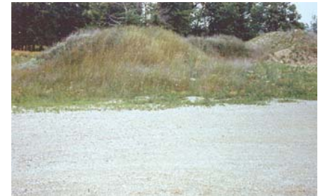
DIRT STOCK PILES—GOOD
