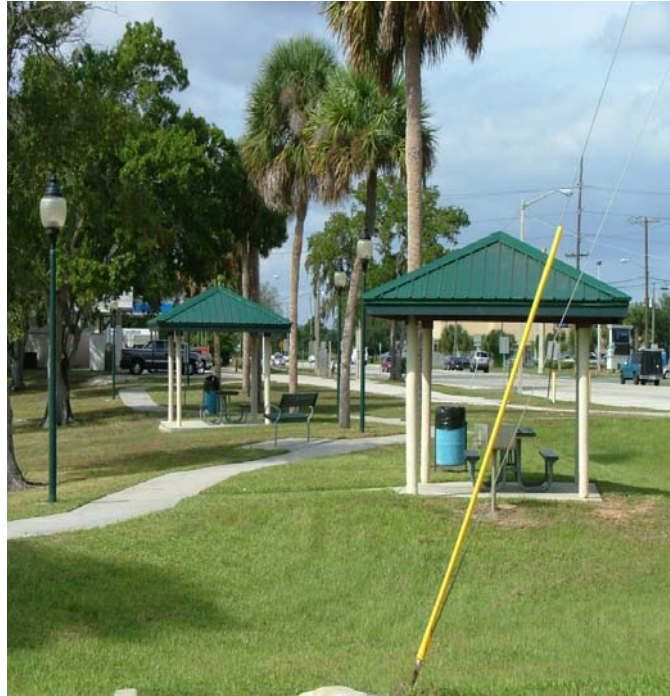
NEW PAVILION ROOFS INSTALLED BY STAFF AT JIMMY MOORE PARK
