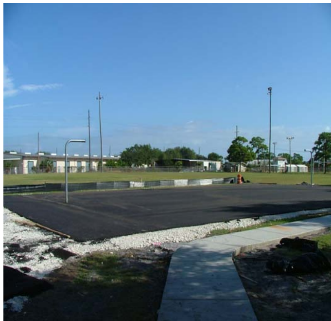
CONSTRUCTION OF NEW OUTDOOR BASKETBALL COURT AT CARVER PARK
